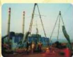
Drilling for Piezometer and inclinometer Installation
